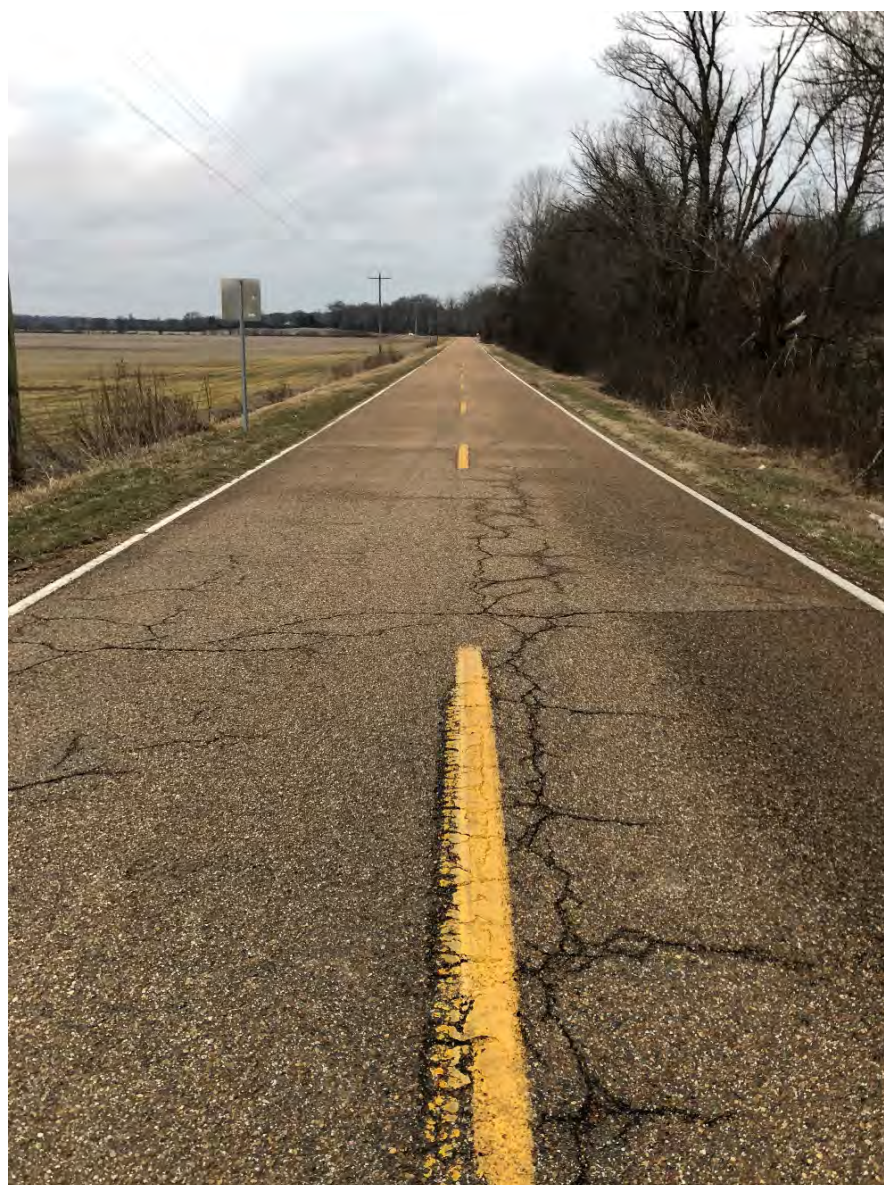
Looking West From Bridge
