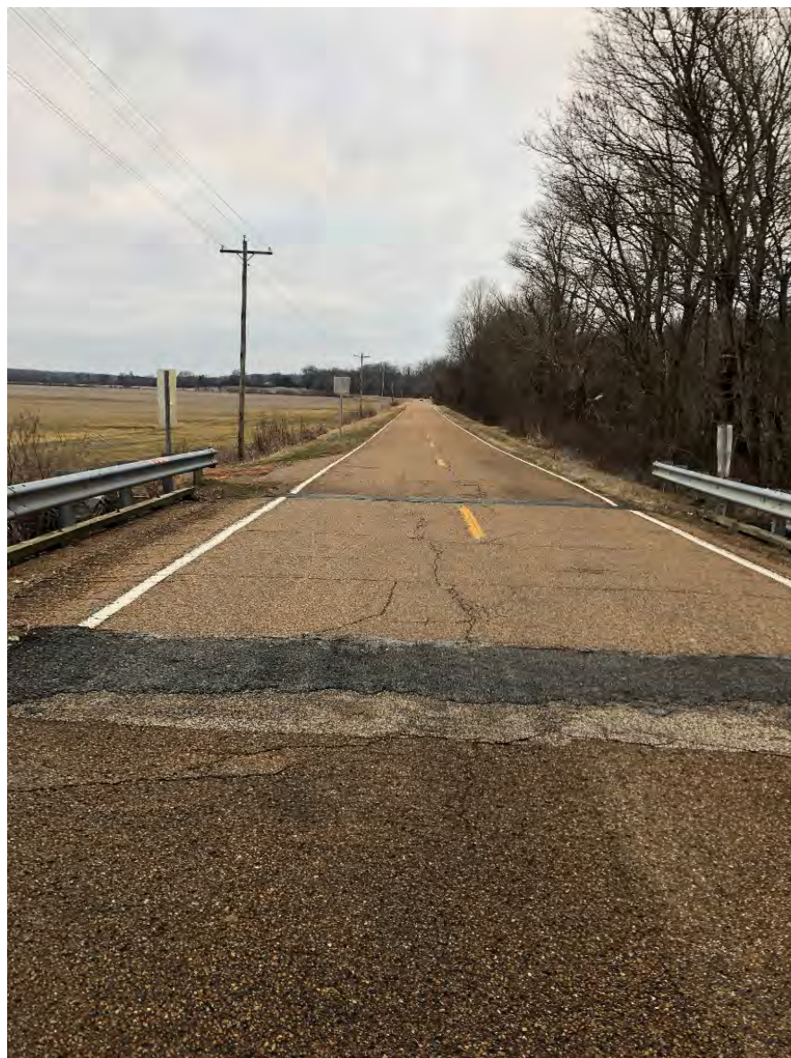
East Approach of Bridge Looking West
