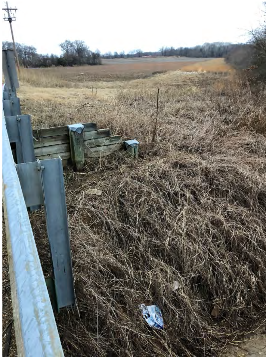
Floodplain Left (East) Downstream
