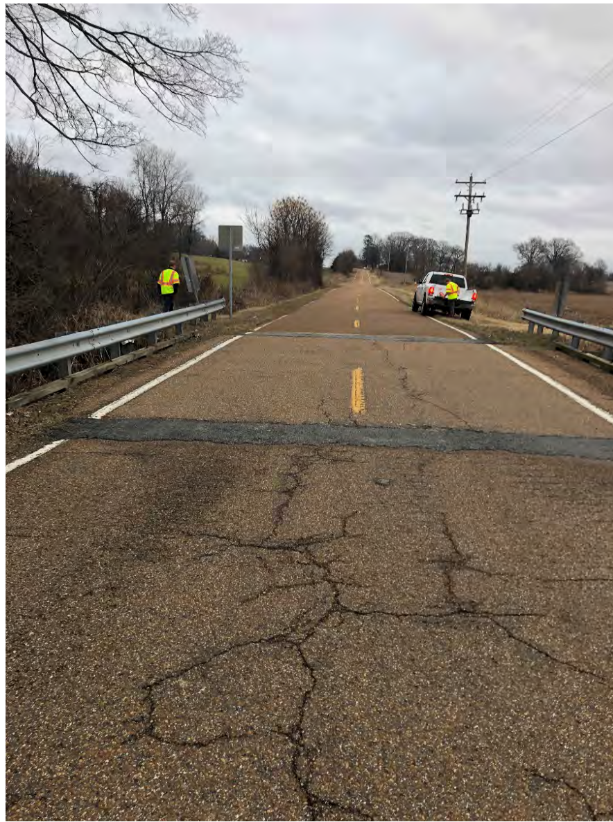
West Approach of Bridge looking East
