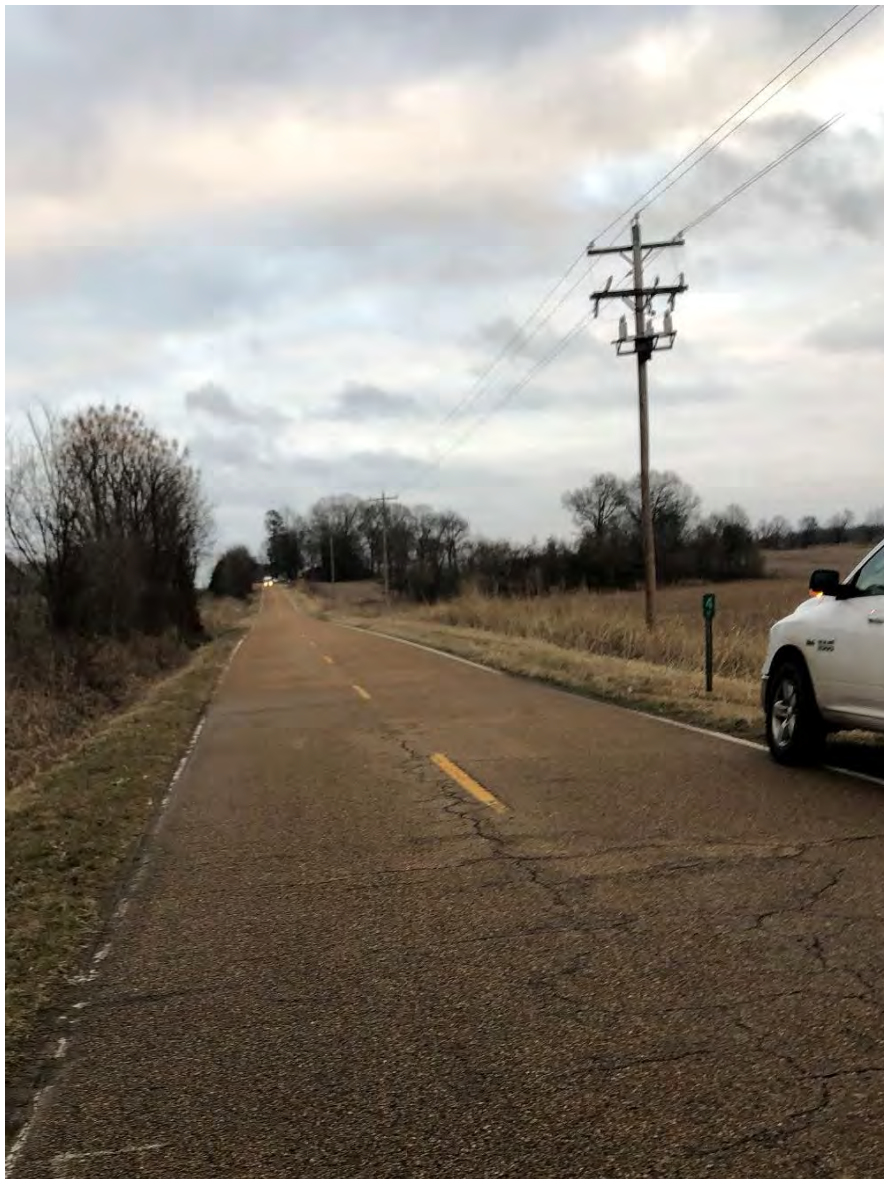
Utility Poles East of Bridge Downstream
