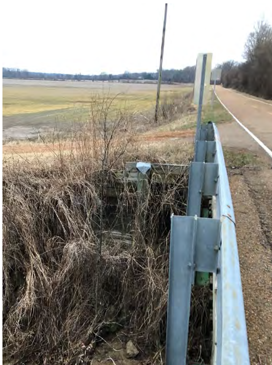
West Abutment at Outlet
