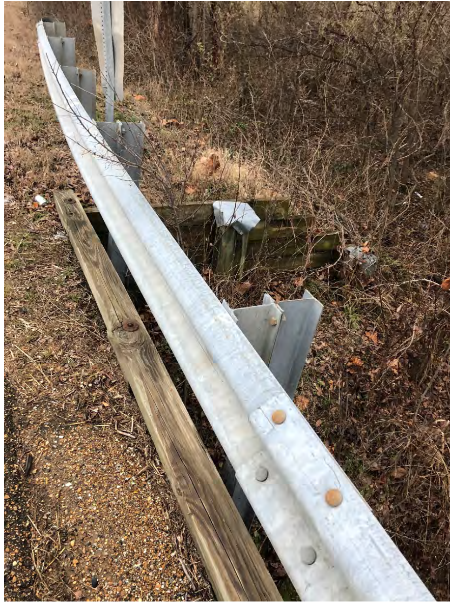
Floodplain Left (West) Upstream
