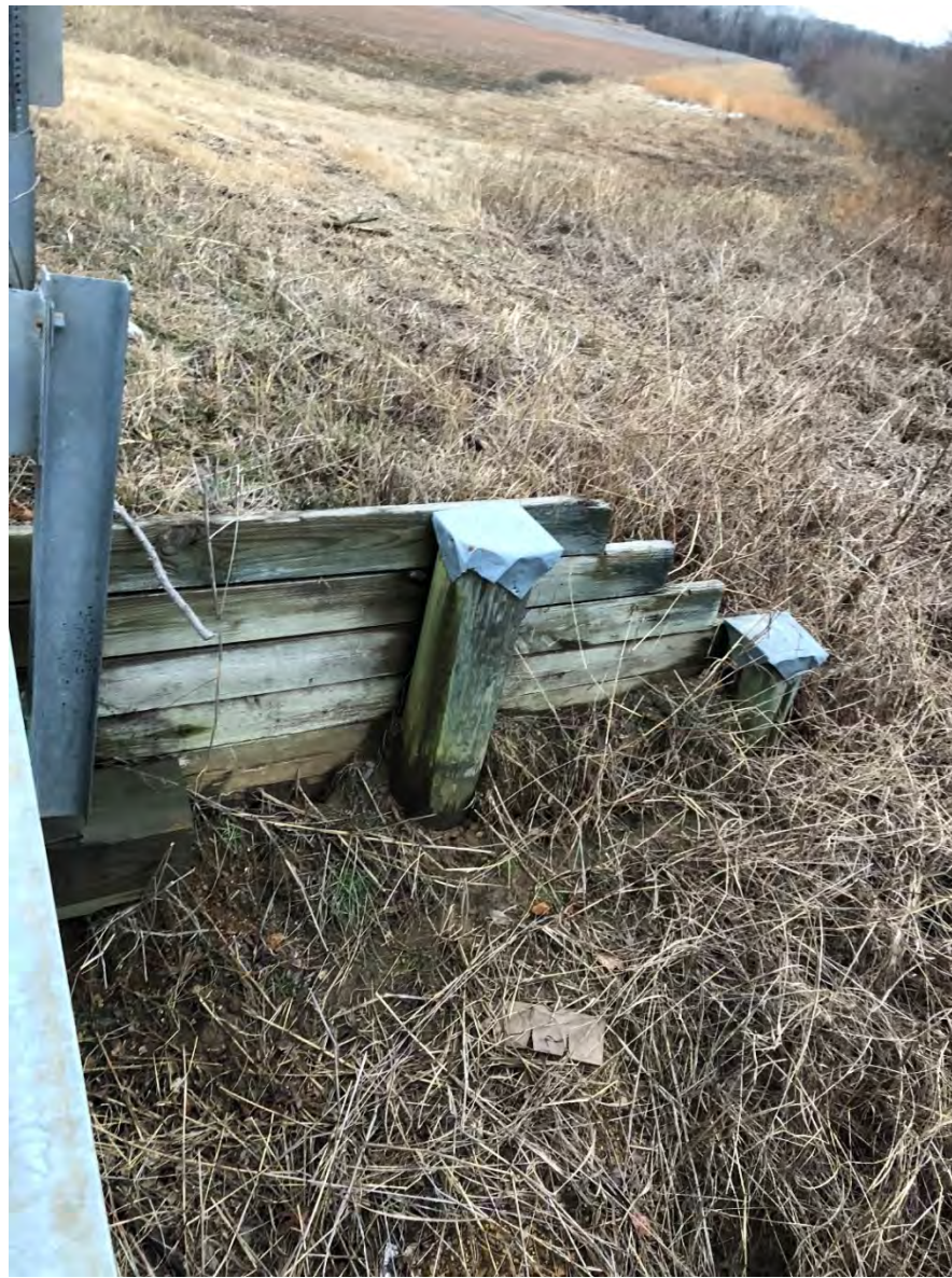
East Abutment at Outlet
